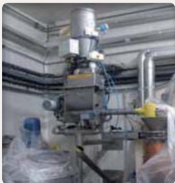
Cyclone transfer system with dosing device
